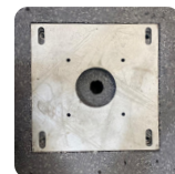
Steel cast in place sign bracket
