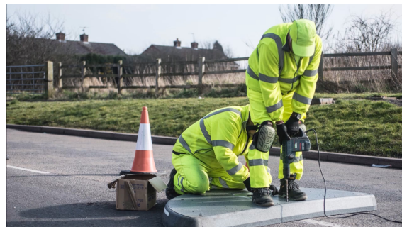
Drill and anchor in place
