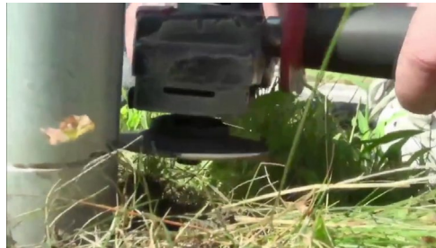
1. Cut damaged post
