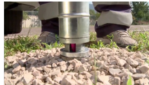
4. Spin SmartFlex into ground sleeve & upper pole
