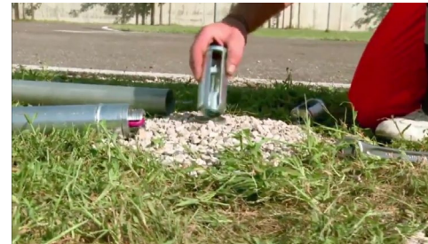
2. Insert expander into ground sleeve
