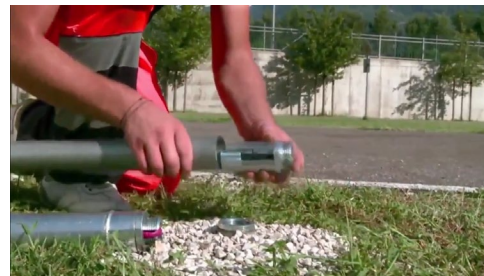
3. Insert expander into upper pole
