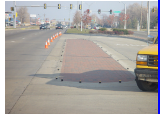
35 Amber Curb Markers installed on a semi raised median with beveled edges . Installation time: 3 Hours
