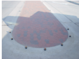
35 Amber Curb Markers installed on a semi raised median with beveled edges . Installation time: 3 Hours
