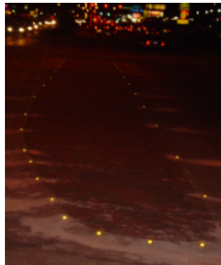
35 Amber Curb Markers installed on a semi raised median with beveled edges . Installation time: 3 Hours
