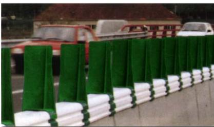
Anti-blinding screens with a fixed angle feature greatly reduce blinding glare, including distractions on the opposite side of the traveled way.
